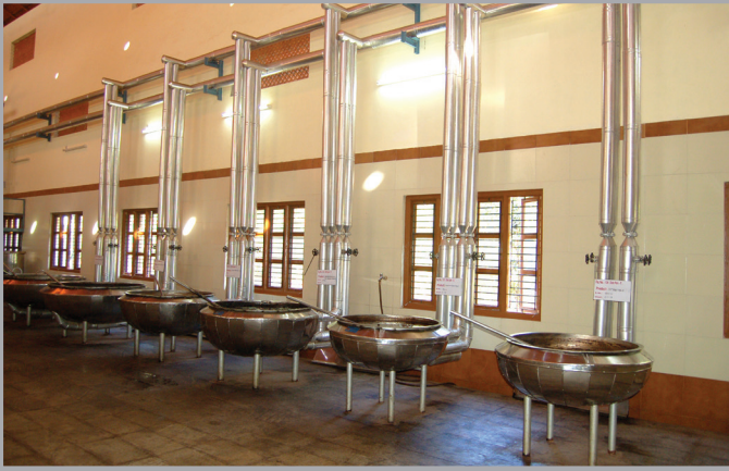
Steam / Thermic Fluid Jacketed pan Arrangement
