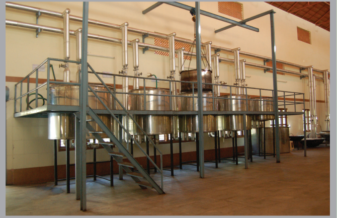
Steam / Thermic Fluid Coiled Drug Boiler Arrangement
